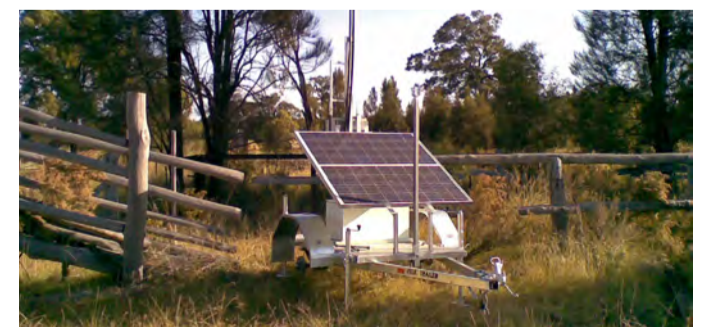
Noise monitoring unit.
