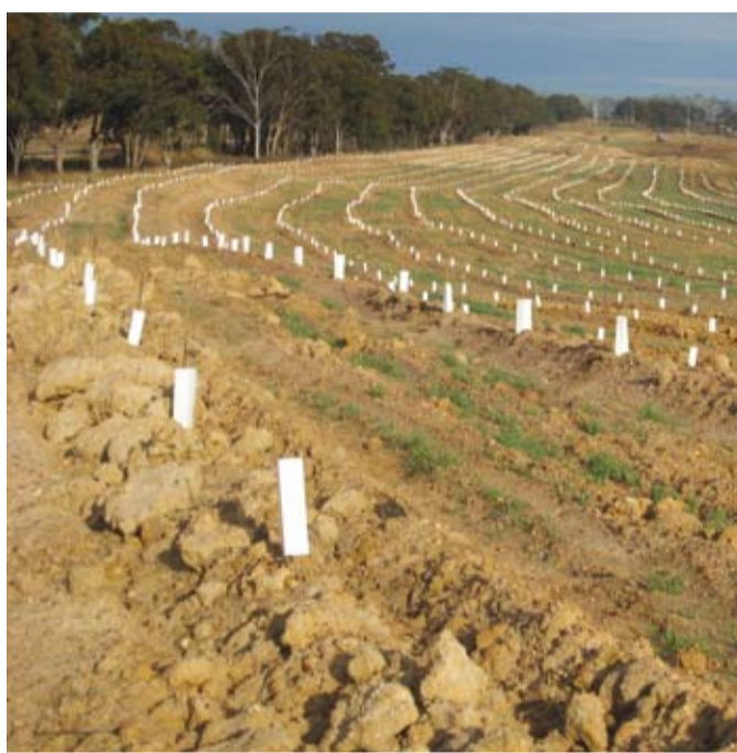
New tree screen area.
